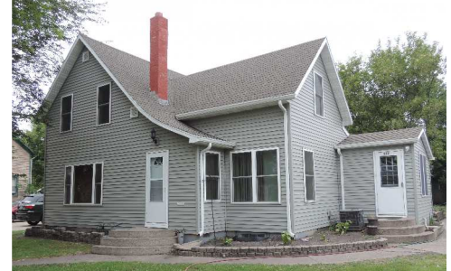
After: New siding, shingles, windows & doors
