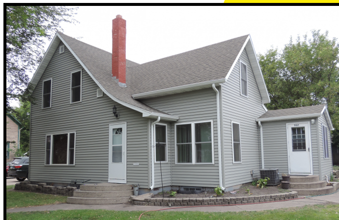
After: New siding, shingles, windows, and doors
